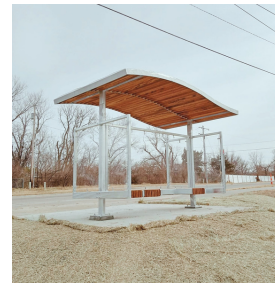
Manhattan Ave. Shelter Completed Jan. 2023
